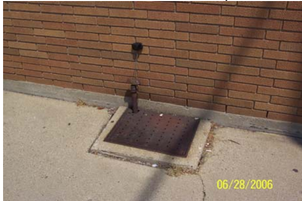
DT 59 – Potential UST Vent Pipe
